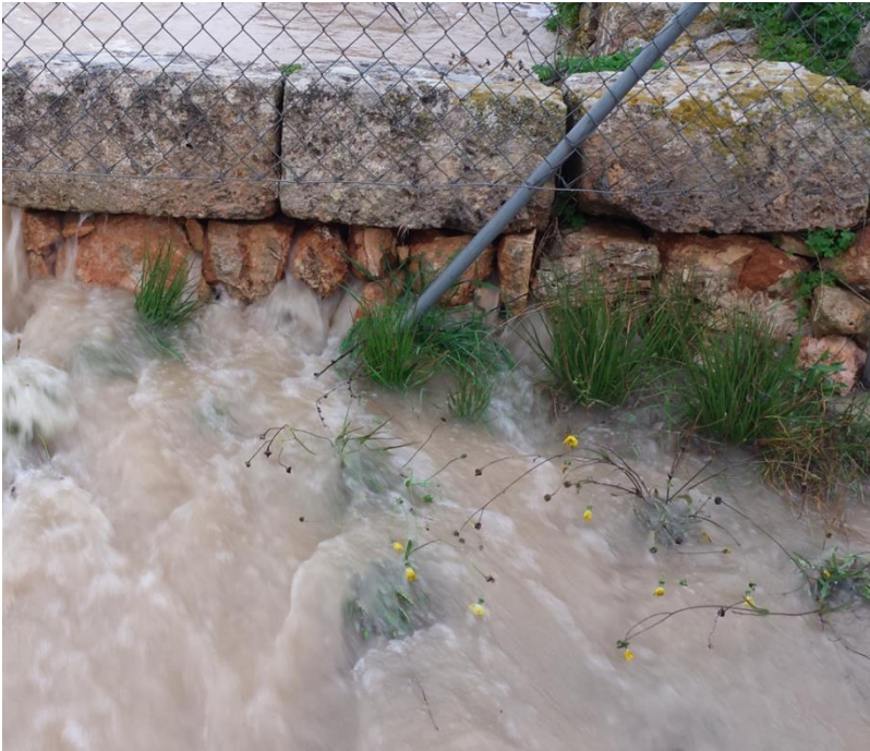
Figure 3 - Wall with holes, allowing the water flow through the stones. Campos Basin, January 2017. Source: Author's research.
